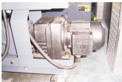
Picture 3-6: Installation of Gear Motor and Coupling
