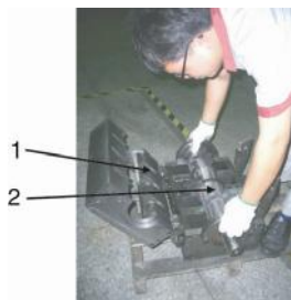
Picture 3-4: Installation of Bearing and Blade Rest 2
