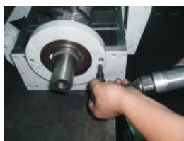
Picture 3-5: Installation of Bearing and Blade Rest 1 3
