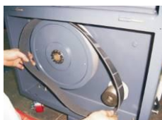
Picture 3-16: Installation of Belt and Belt Pulley 6
