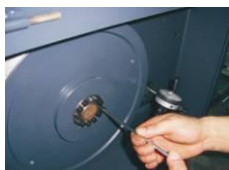
Picture 3-14: Installation of Belt and Belt Pulley 4
