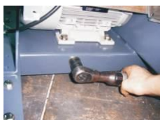
Picture 3-18: Installation of Belt and Belt Pulley 8
