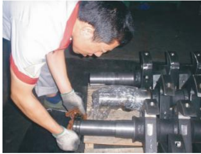
Picture 3-3: Installation of Bearing and Blade Rest
