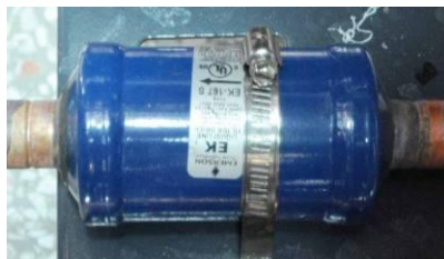
Picture 2-6: Drying Filter
