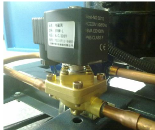
Picture 2-10: Liquid Pipe Solenoid Valve
