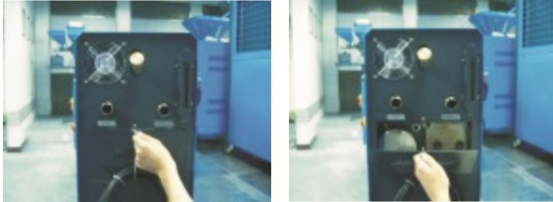
Picture 6-9: Cooling Pipes 1
