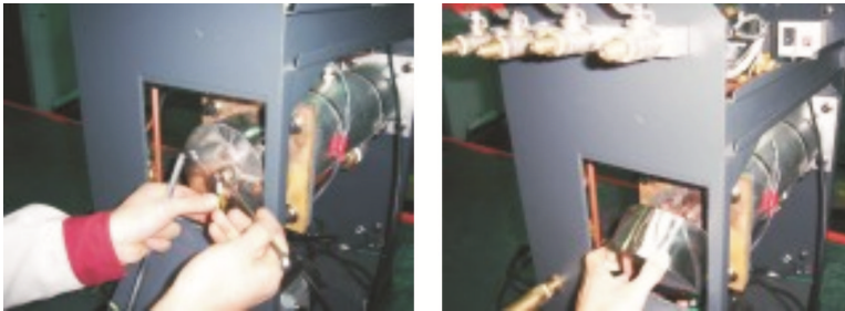
Picture 6-7: Pipe Heater 2
